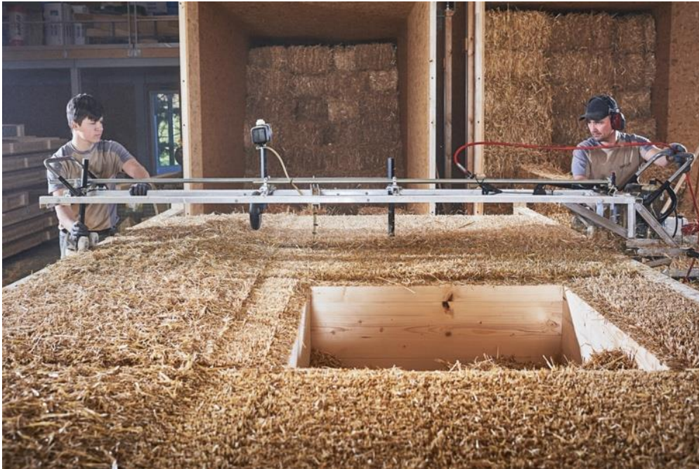
Figure 12. Prefabrication of wall modules for Bombasei. Photo: Damian Poffet, 2019
