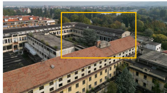
Figure 3. Part of the ex Manifattura Tabacchi. In the yellow rectangle, the building object of study.
