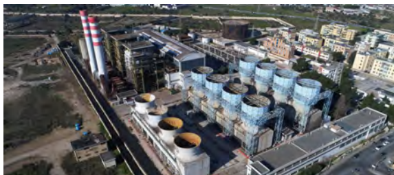
Figure 1 The ex-thermoelectric power plant of Bari (see online version for colours)
