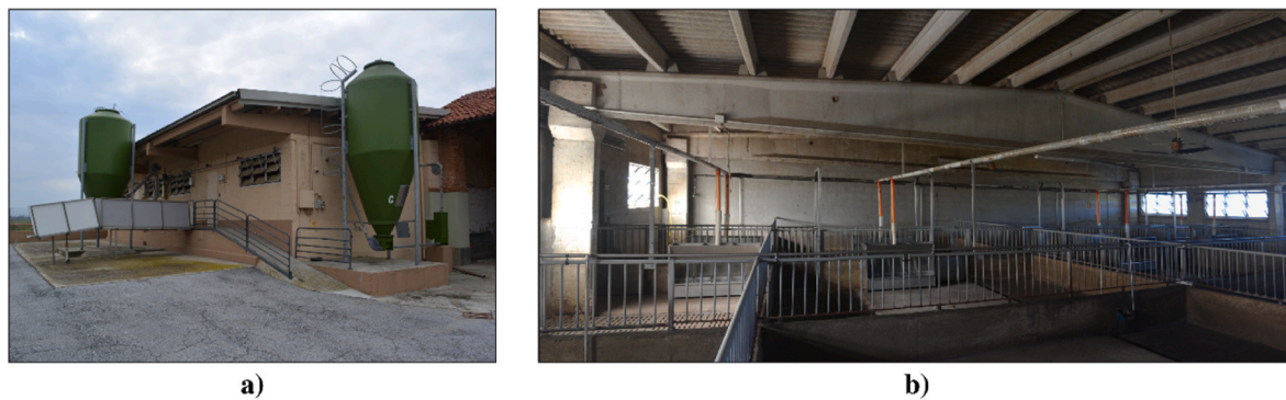
Fig. 3. External (a) and internal (b) views of the analyzed pig house.
