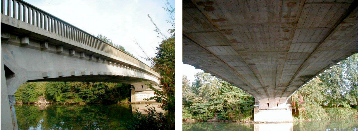
Figure 2 (a & b) Views of the Luzancy Bridge by E. Freyssinet 1946 (Courtesy of www.structurae.net ).
