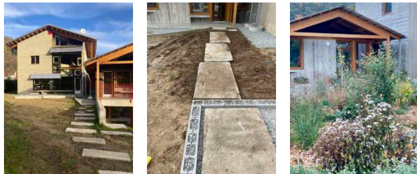
Casa BM, the cataloguing and reuse of materials from the site and its immediate surroundings. Steps from the demolished staircase of the original building define the paths around the house, while stone slabs from a nearby ruin mark the entrance area. The garden forms a patchwork of 'domestic' and 'wild' plants—some purchased, some preserved, others arrived by chance or found along the roadside. Photo: ErranteArchitettura
