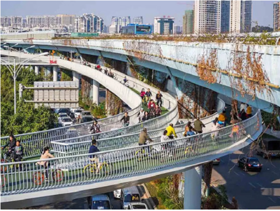
Figure 1.33. A transformation towards sustainable mobility indispensably implies an infrastructure dedicated to cycling that offers safety in all aspects. Source: https://ciclosfera.com/a/skyway-puente-ciclista-largo-mundo-xiamen
