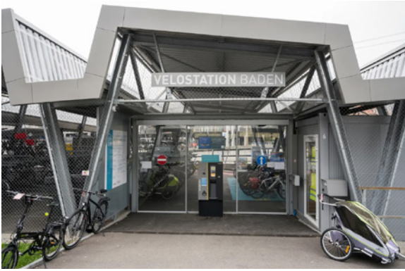
Figure 1.56. The Velostations are a style of architecture that encourages bicycle riding while simultaneously supporting intermodality. Source: https://www.aargauerzeitung.ch/aargau/baden-270-zusaetzliche-veloparkplaetze-beim-bahnhof-ld.2161972
