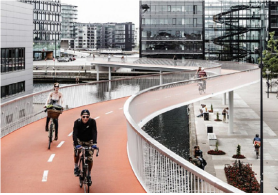
Figure 1.29. Dissing + Weitling. (2014). Cykelslangen. Source: https://www.climateaction.org/news/germany_is_building_worlds_biggest_bicycle_highway
