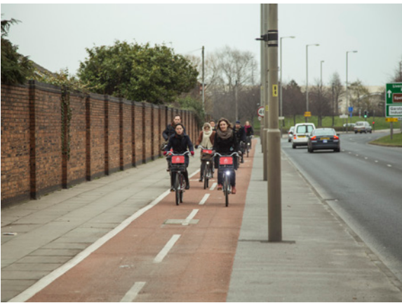
Figure 1.34. It is perfect for separating motorized traffic from bike lanes and traffic carried by cyclists and pedestrians. Giving each form of displacement space would be the wisest course of action. Source: https://www.flickr.com/photos/16nine/16246112923/in/album-72157657144439151/
