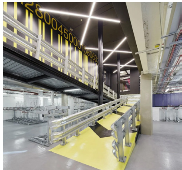
Figure 1.54. The bicycle architecture must have a configuration that allows continuity in movement, leaving and entering the building without getting off the seat if desired. Source: Studio RHE. (1026). Alphabeta Building .
