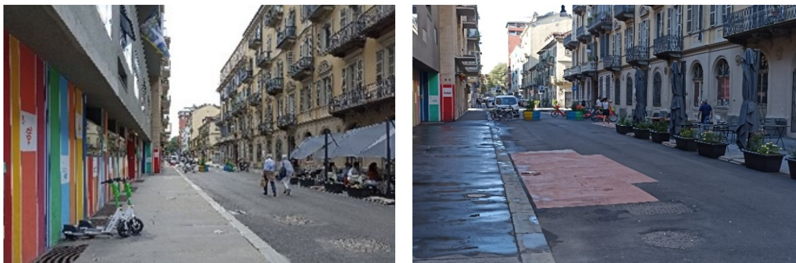
Fig.3 Principe Tommaso Street in the temporary (on the left) and permanent (on the right) version
