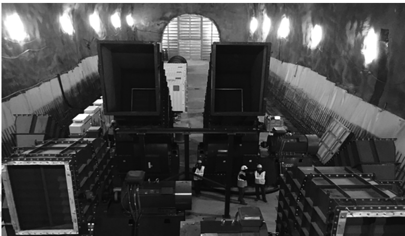
Figure 6.57 Centrifugal fans during installation.
