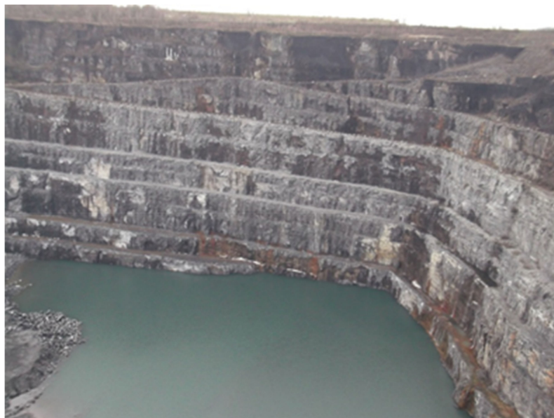
Figure 1. Open pit lake, with raising water level in the basin, ready for backfilling (credits C. Oggeri).
