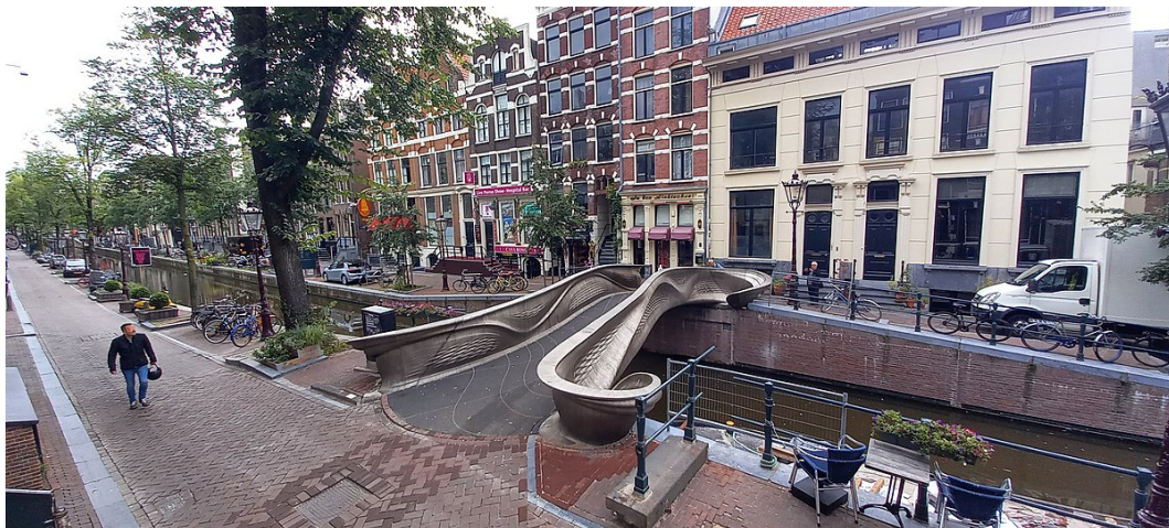
Fig. 1.1 MX3D bridge, world's first 3D printed stainless steel bridge in Amsterdam (NED)
