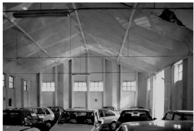
Fig. 12: Pier Luigi Nervi, Ferrocemento prototype in via della Magliana, Rome, 1945. View of the interior (2017, photo by Fondi)
