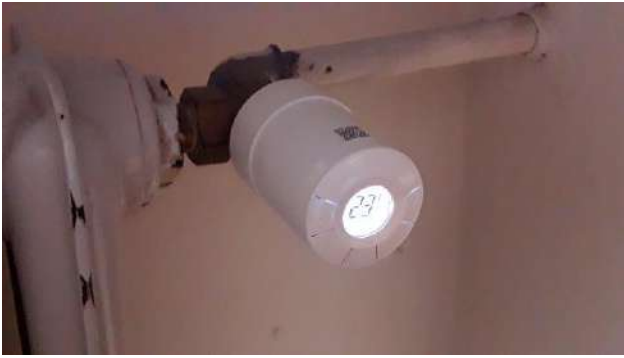
Fig. 7: Installed actuator (thermostat)
