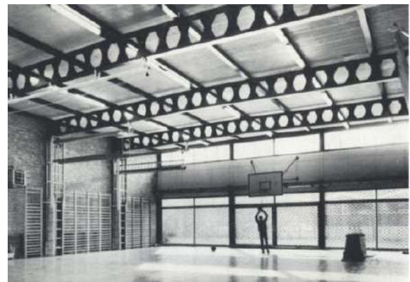
Fig. 2: Photo of the building, made by F. Niffle. 4
