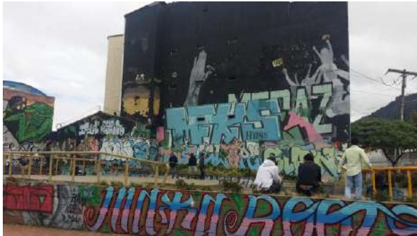
Fig. 5: The area of the 'Avenida 26' occupied by skaters. In the background, one of the municipally-sponsored public art, now covered with tags
