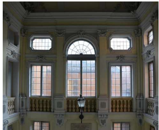
Fig. 18: Staircase, view from the second landing towards the back wall with the serliana
