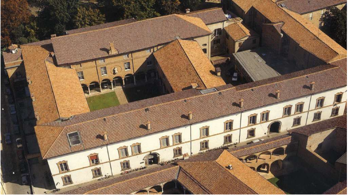
Fig. 1: The complex of Estense Gavassini Pareschi palace
