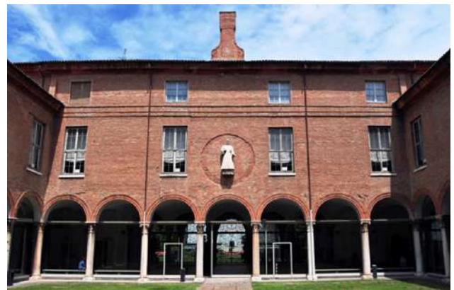
Fig. 13: Photo of the northern block front by the inner
