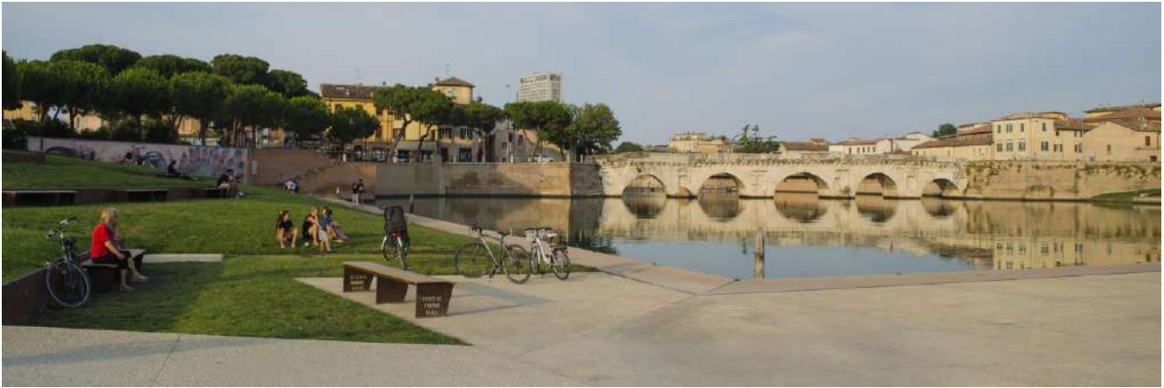
Fig. 10: The bridge view from the platform next to the water basin.
