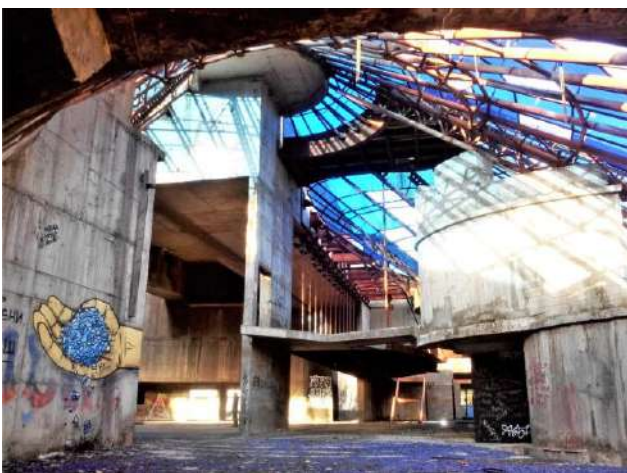
Fig. 17: Interior spaces, today
