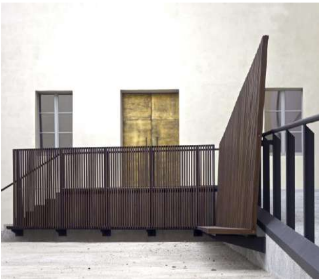
Fig. 16: the entrance ramp and wooden bench - Ph. A. Chemollo
