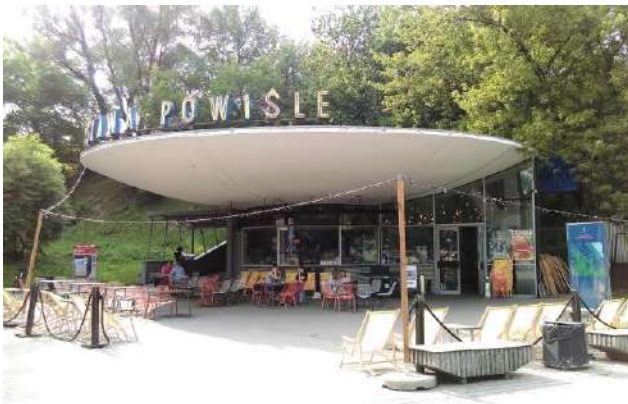
Fig. 2: PKP Powisłe Cross-City Line railway station. The old ticket office pavilion became one of the trendy cafeterias in Warsaw. Architects Arseniusz Romanowicz and Piotr Szymaniak, 1963. (photo of the author, 2017)
