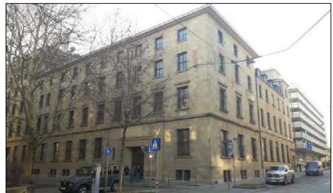
Fig. 2: Building 2 of HFT Stuttgart
