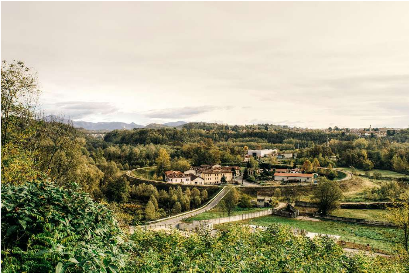
Fig. 2: View of Mulini di Gurone (VA), surrounded by the circular dam, 2017.
