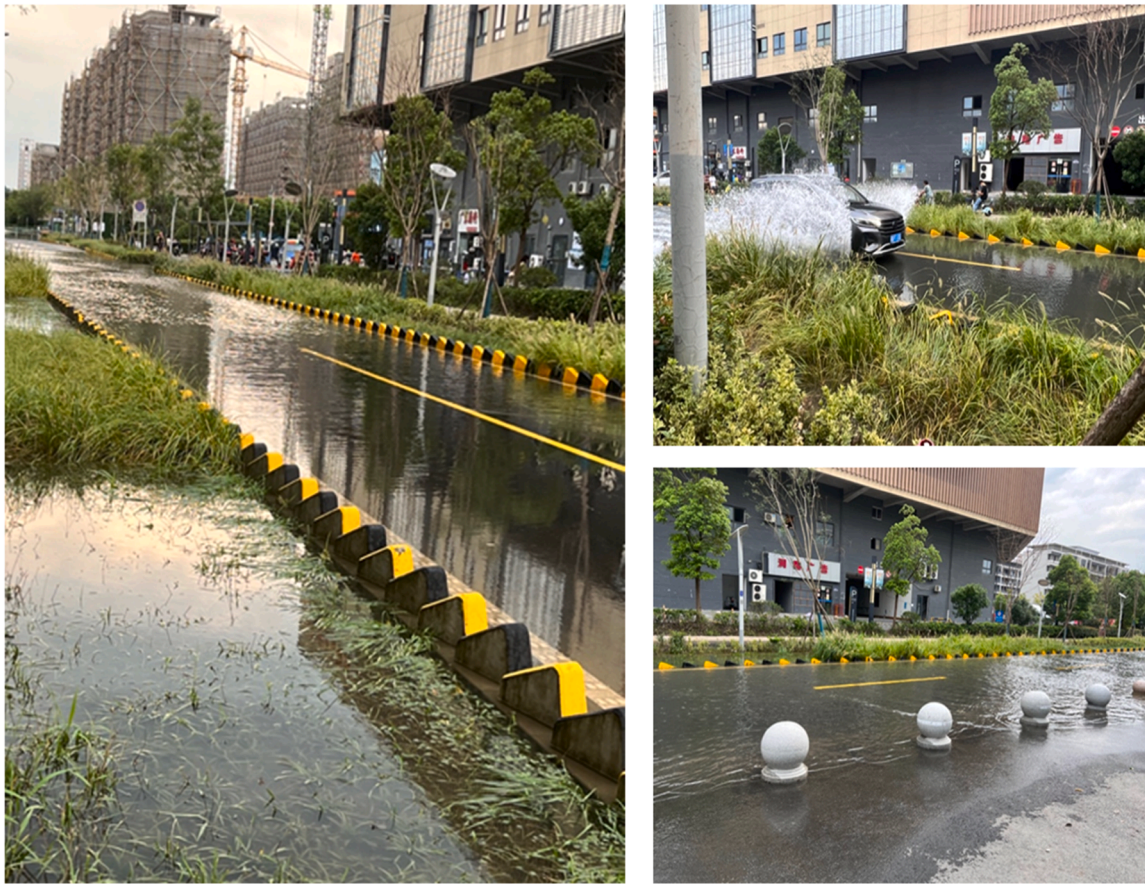
Fig. 3. Flood occurrence after typhoon Muifa on 13 September and inundation of the swale. Photo source: Lingwen Lu (approved to use the photos). (For interpretation of the references to color in this figure legend, the reader is referred to the web version of this article.)
