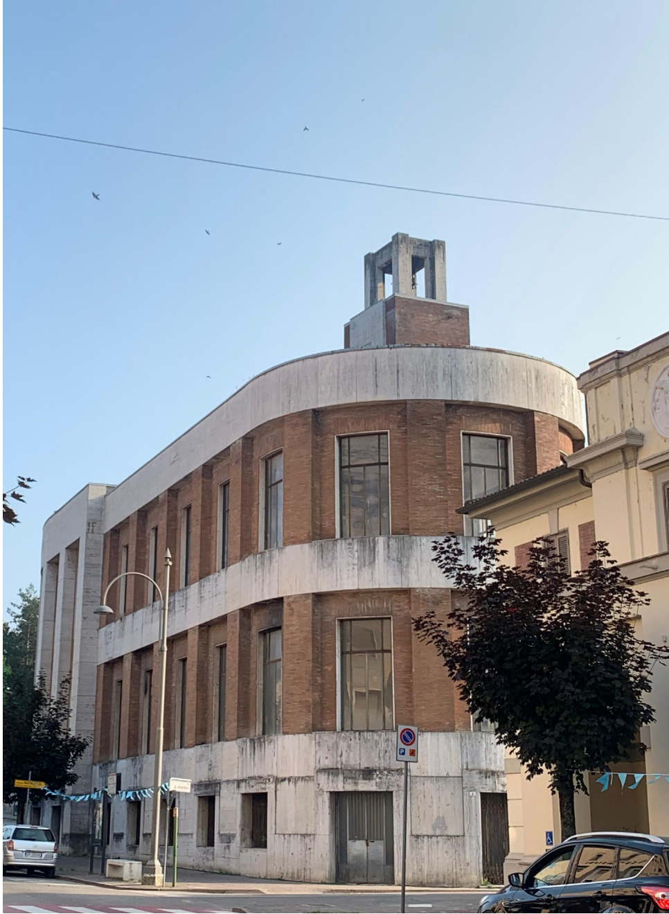
View of Former House of the Fascist Party, Predappio, Italy, June, 2025
