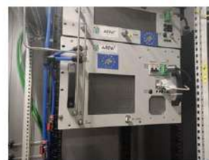
Figure 2 Installed electrolyser at ZEM module
