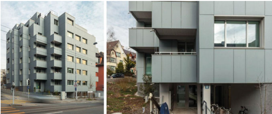
Fig. 29.12 Renovation of an apartment building
