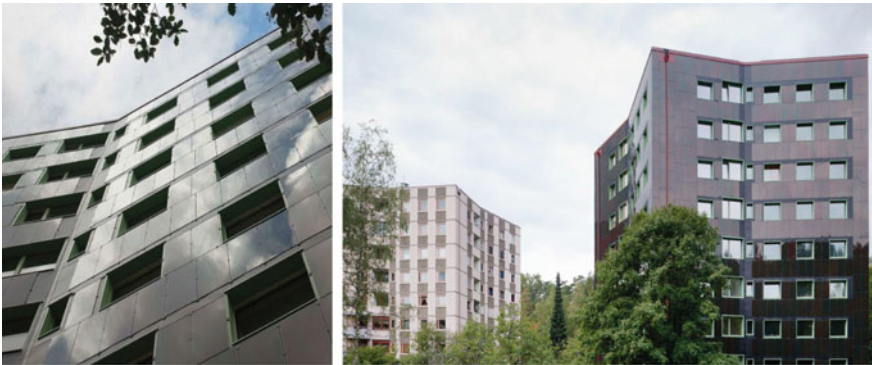
Fig. 29.13 Renovation of Stacken apartment building
