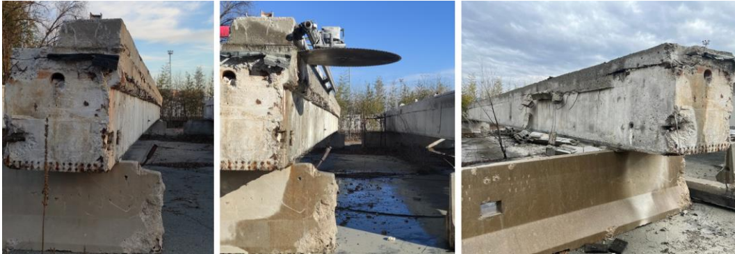
Figure 42: Working phases of curb cutting.
