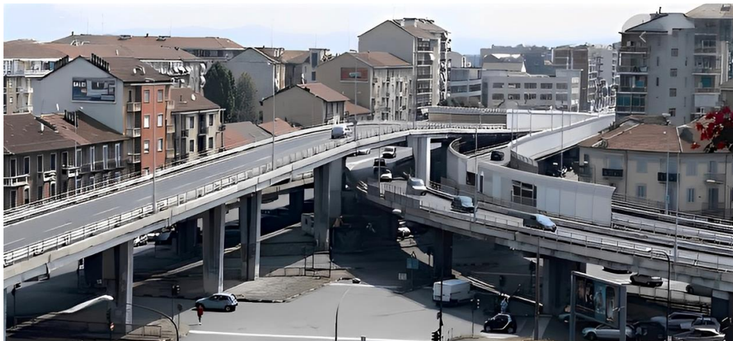
Figure 1: C.so Grosseto viaduct (west view).
