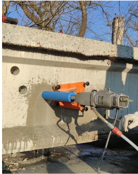
Figure 53: Concrete coring.
