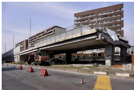
Figure 10: End parts tested within the BRIDGE|50 research project.
