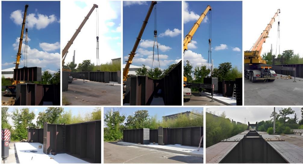
Figure 24: Building stages of the steel reaction frame.
