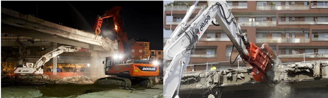
Figure 9: Demolition of the bridge using hydraulic crushers.
