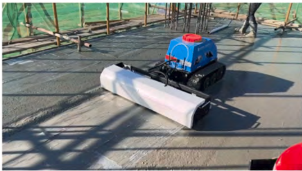
Fig. 15. Robot plastic film curing operation.
