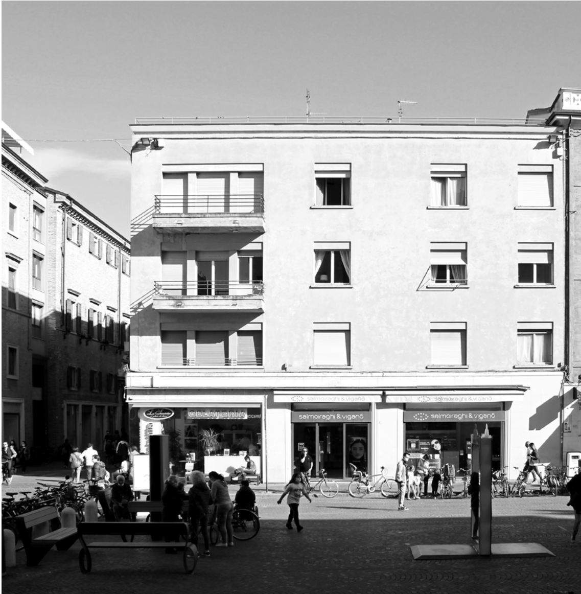
Fig.8 – Example of a building that respects the block morphology but presents modernist canons. Piazza Cavour, 1, 47921 Rimini RN. Picture. Source: Author, 2020
