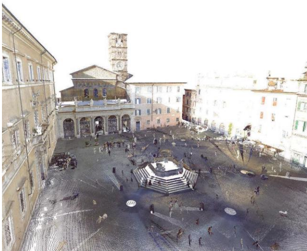
Figure 5. The Basilica of Santa Maria in Trastevere, numerical model from the elaboration of 3D laser scanner survey.
