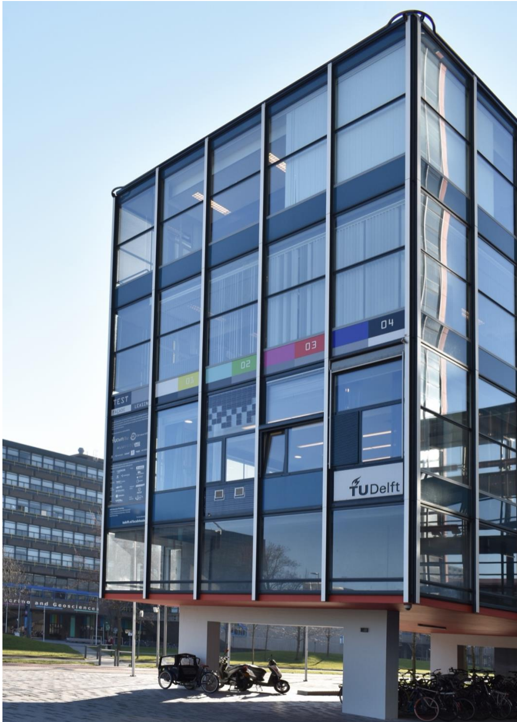
Figure 33: Façade Leasing prototype at TU Delft campus university
