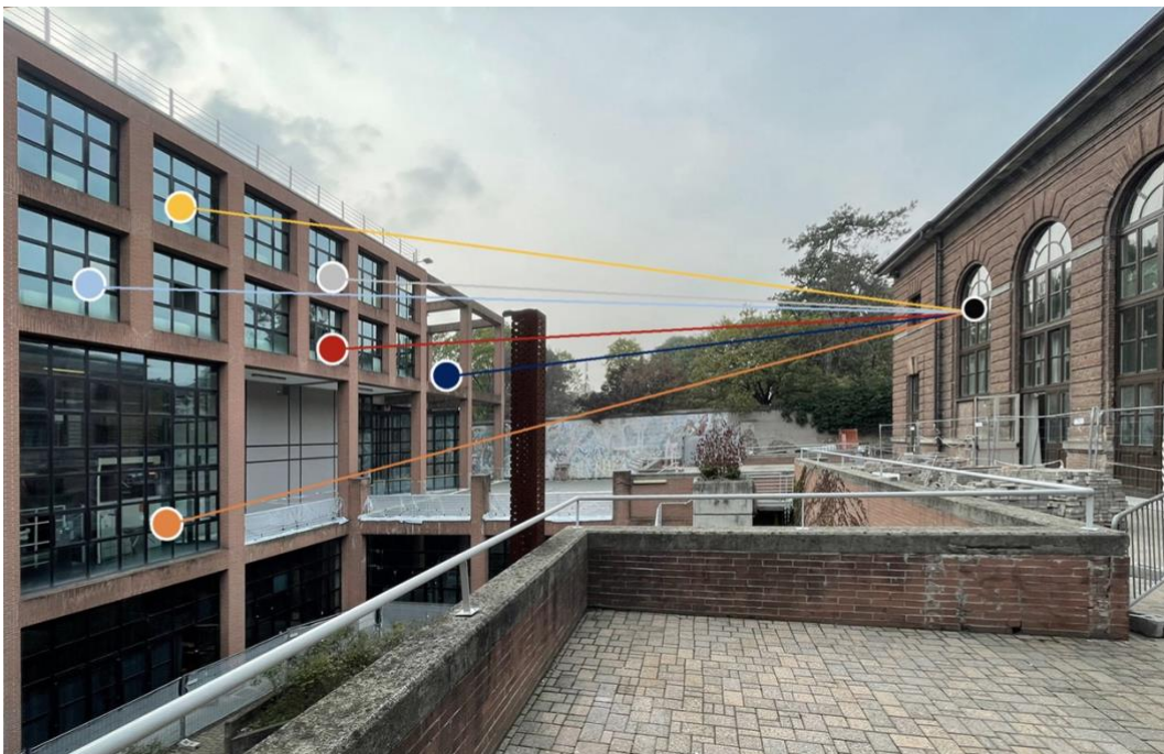
Figure 45: RFI sensor grid installed. In the building on the right was placed the antenna
