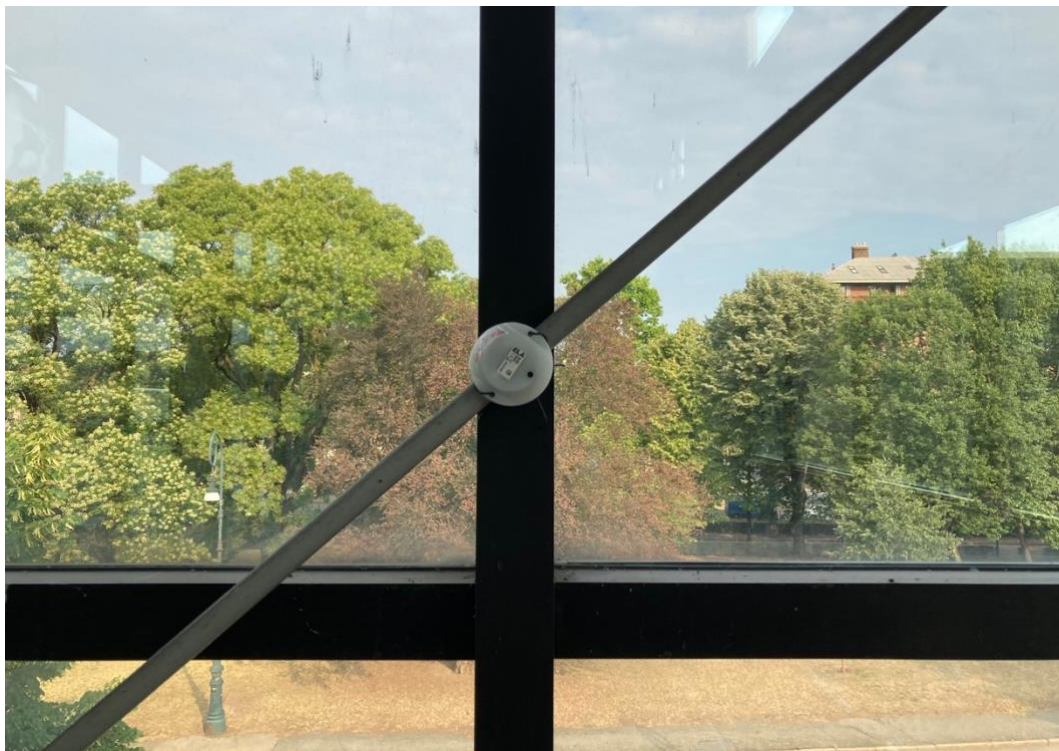
Figure 44: RFID sensor installed on the internal façade during the first campaign monitoring
