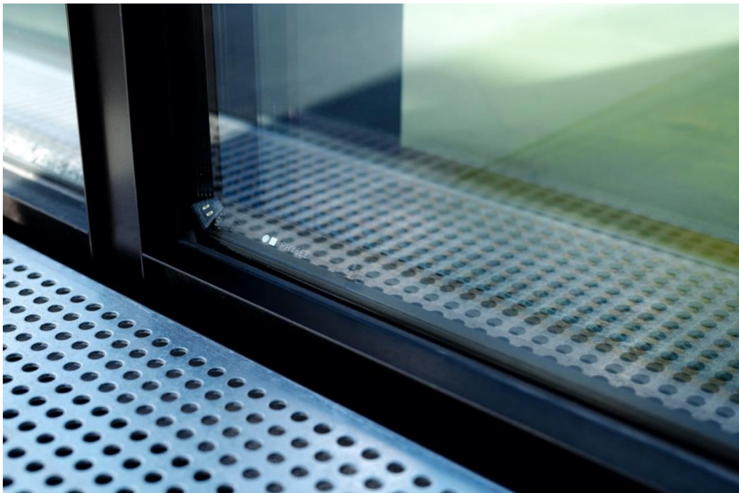
Figure 36: Physee SENSE - Smart Window (credit: Timbuiting).
