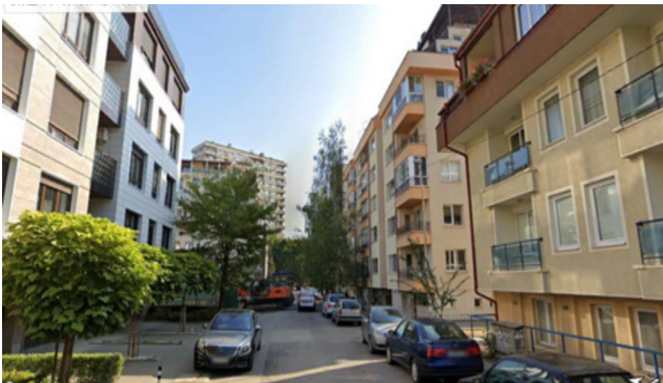
Middle Class housing in Bulgaria. Krasno selo residential estate in Sofia, 2019 (@Google Earth Pro)
