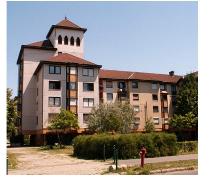
Gloriette housing estate built in the second half of the 1980s in the 18th district of Budapest (© Tamás Egedy, 2017)
