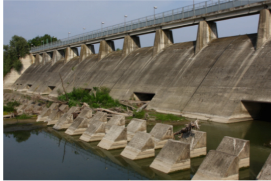
Fig. 1. Flood dam of the Sant'Anna flood control reservoir [4].
