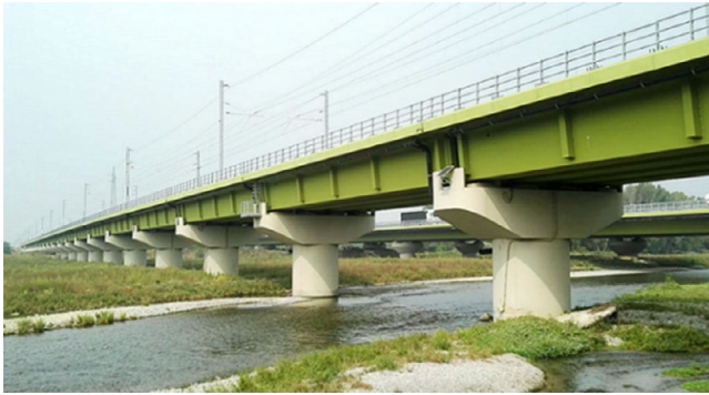
Figure 1. View of the Oglio Viaduct.
