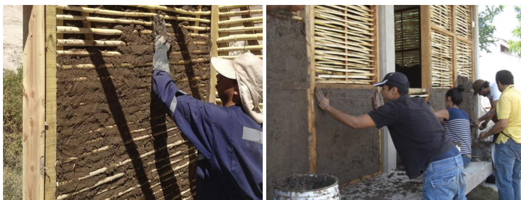
Figure 62. Examples of traditional earthquake-resistant construction techniques: Quincha 129 wall, used in Chile and Peru (left); Bahareque wall, used in Colombia and Venezuela (right).
