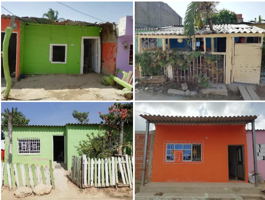
Figure 102. Four of the ten self-built houses analyzed in El Pozón.
