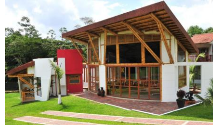
Tendinous System: it fuses wattle and daub architecture, to which barbed wire is added for tension and sacks and mats filled with cement. Casa Montoya / Carolina Zuluaga Zuleta. Fusagasugá, Cundinamarca (CO).
