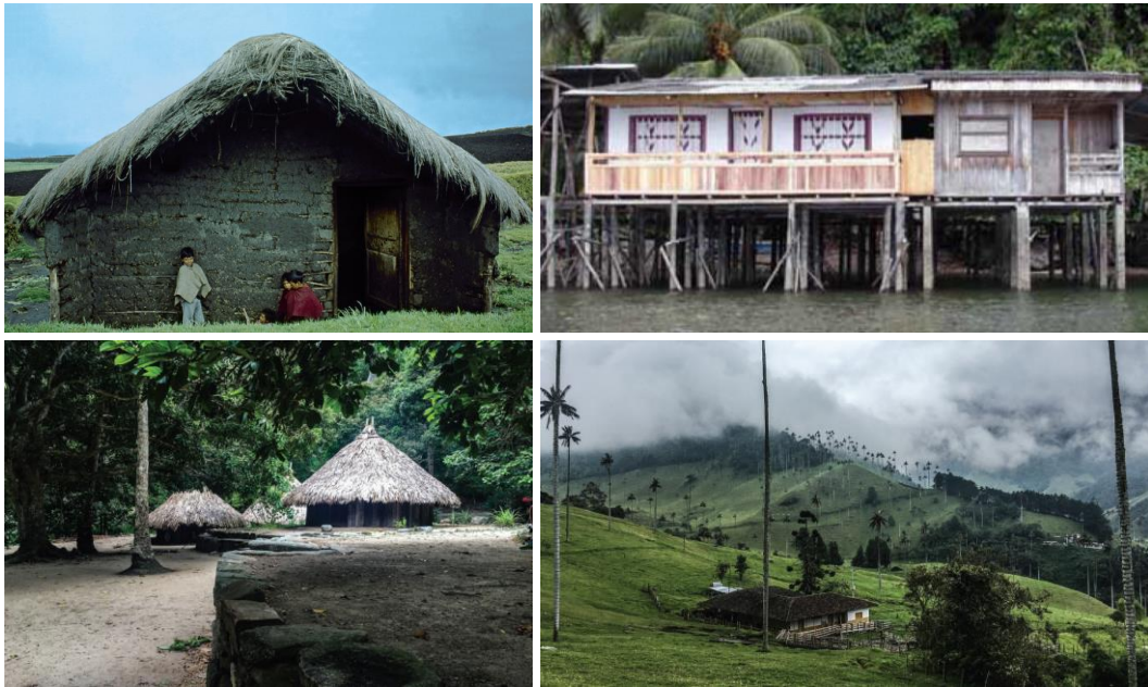
Figure 59. Examples of vernacular architecture: Archetype of a rural house, Nariño, 1979 (top left); Palafitic housing: house in transition to modern in Buenaventura, (top right); Pueblito Chairama - Tayrona National Park , (bottom left); Coffee Cultural Landscape - Cocora Valley , (bottom right).
