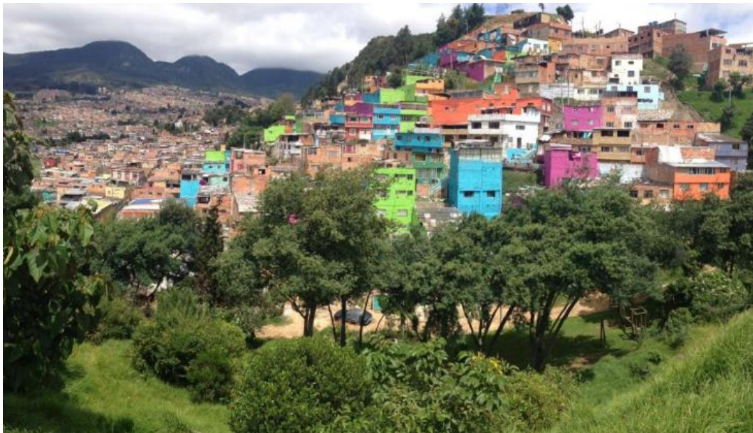
Figure 50. Façades painted by the inhabitants through the “ Habitarte ” program of the Bogotá Mayor’s Office.
