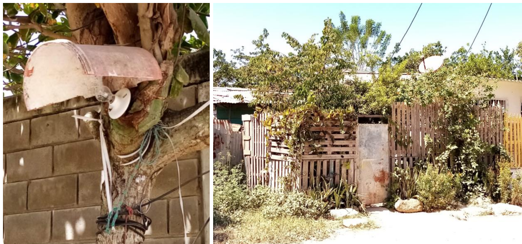
Figure 57. Informal solution to protect street lighting (left) and a fence made of pallets (right).
