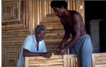
Carpenters working on an interior wall. Huina, Chocó (CO).
