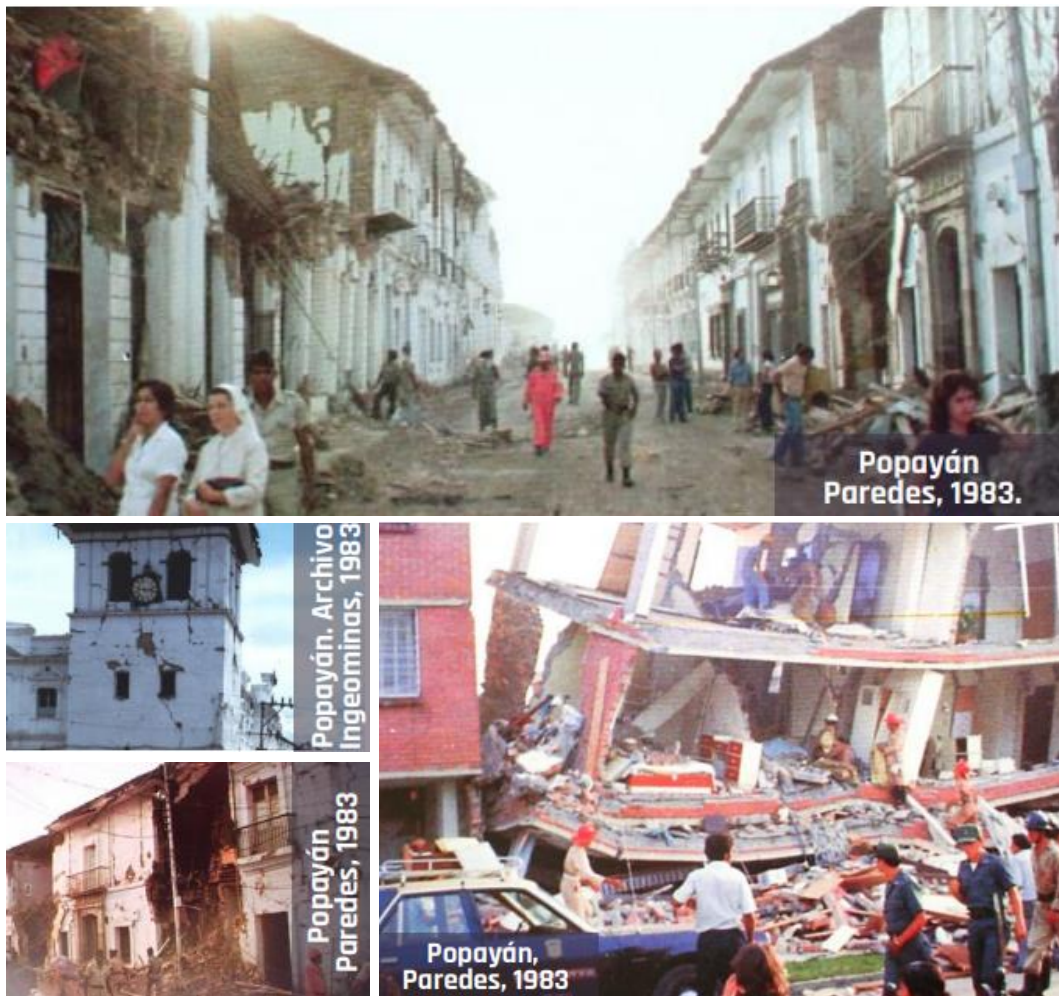
Figure 58. Buildings partially or totally destroyed by the earthquake. Popayán, 1983. Source: https://www2.sgc.gov.co/Archivos/Sismo_31_03_1983%20(11).pdf . Accessed June 1 st , 2022.
