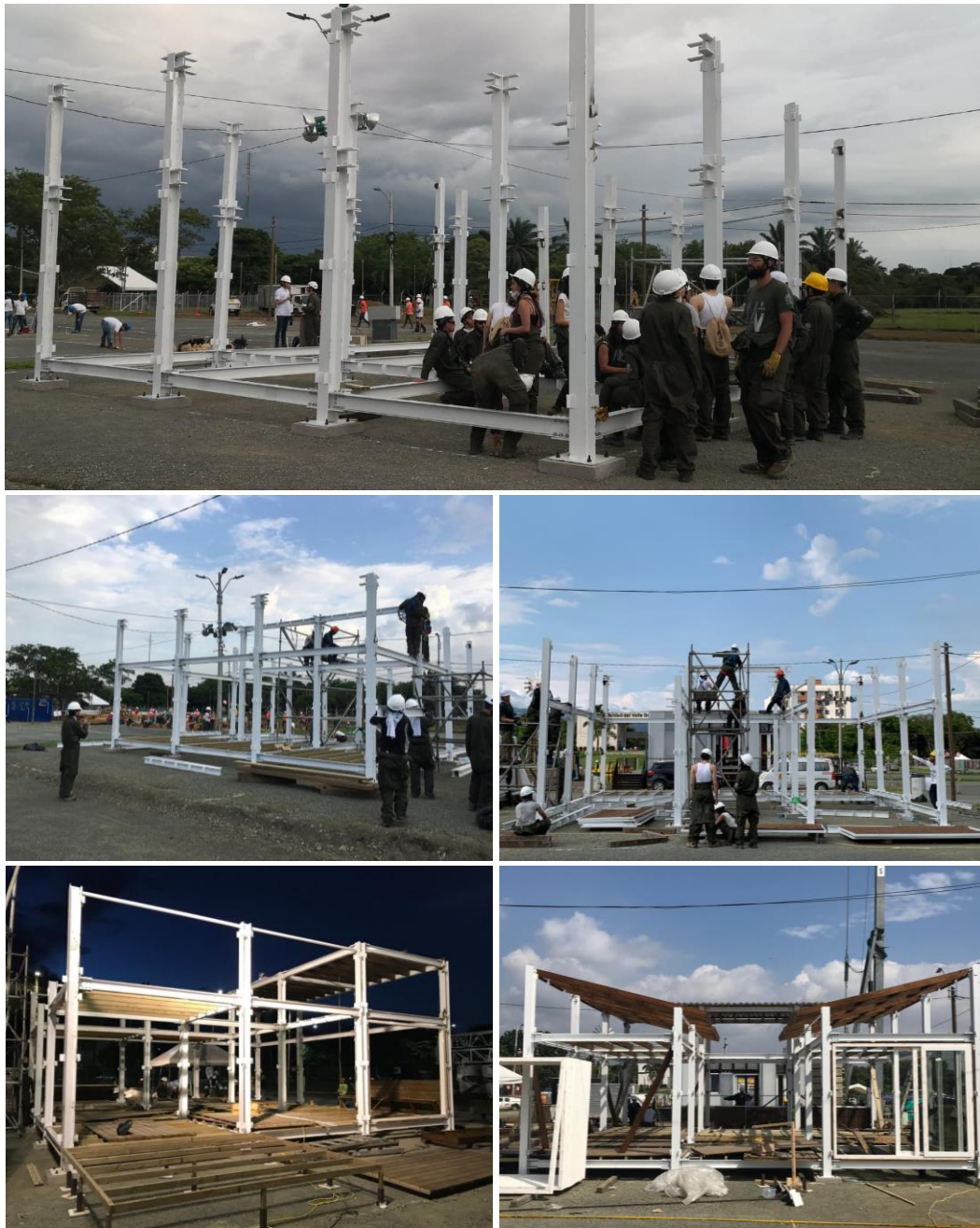
Figure 119. The chassis: steel structure. Source: PEI team, 2019.
