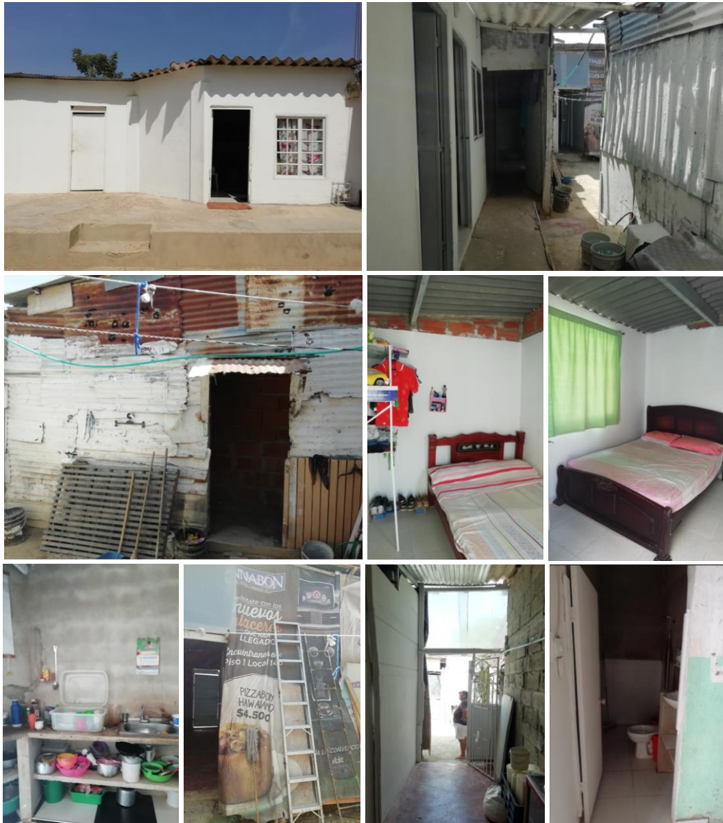
Figure 141. Exterior and interior of Fanny and Hermes' house.
