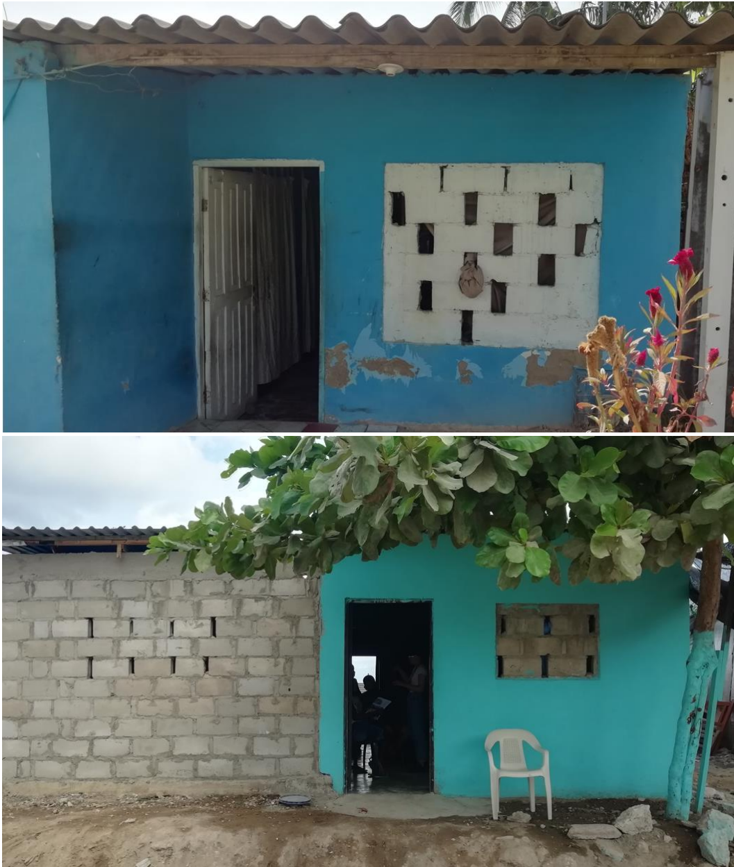
Figure 35. Attempts to make a latticework with concrete bricks to improve internal comfort.
