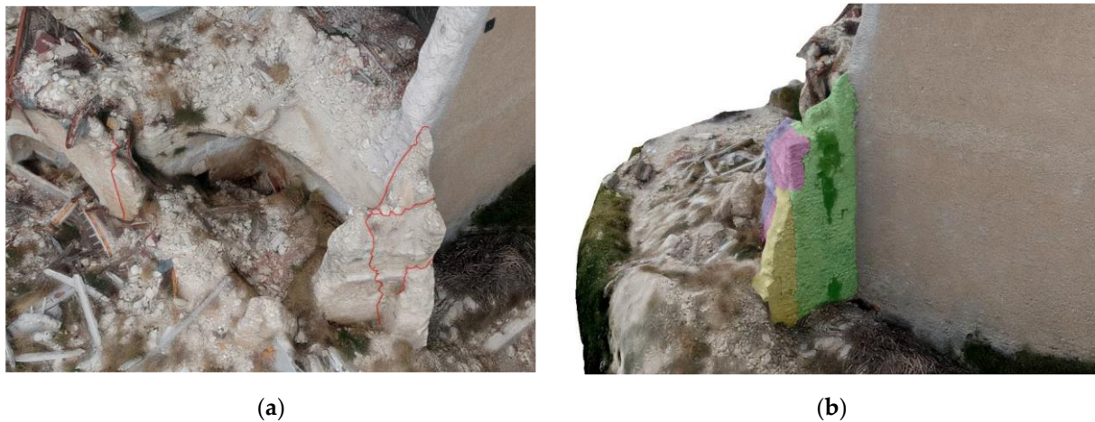
Figure 10. (a) Investigation of the anterior portion through the 3D mesh model textured by HD UAV images. (b) Recognition of the different portions of masonry not clamped or separated by cracks.
