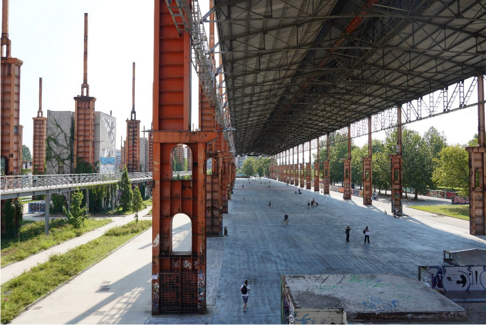
Figure 1) View from South-West of former Vitali's sheds 10 years after the adaptive reuse, designed by Latz and Partners, June 2021, Parco Dora, Turin
