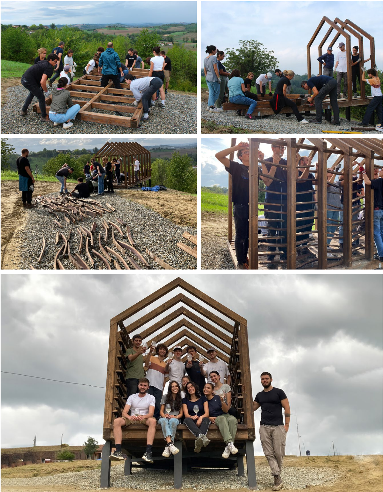
Figure 6 | On-site production phase: above, positioning of the floor beams on the foundations, assembly of the modular portals, anchoring of the barrique walls; below, the completed belvedere.
