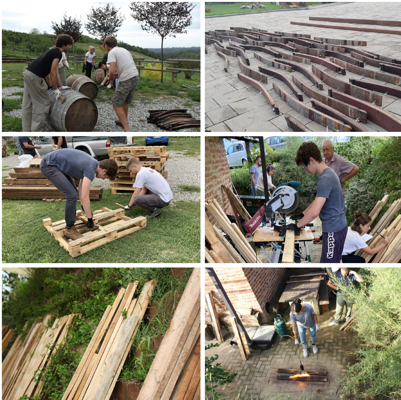
Figure 5 | Some activities of the off-site production phase: above, disassembly of the staves of the old barrels and anchoring on steel cables; middle and below, unnailling, selecting, cutting, and burning the planks recovered from the decommissioned pallets).
