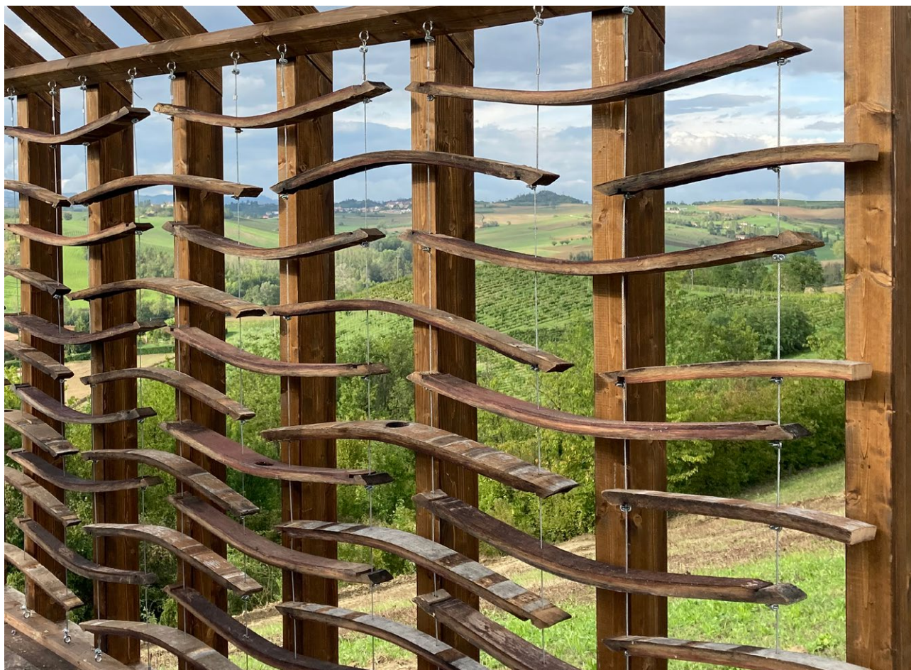
Figure 7 | Detail of the connections between barrel staves, steel cables and structure.
