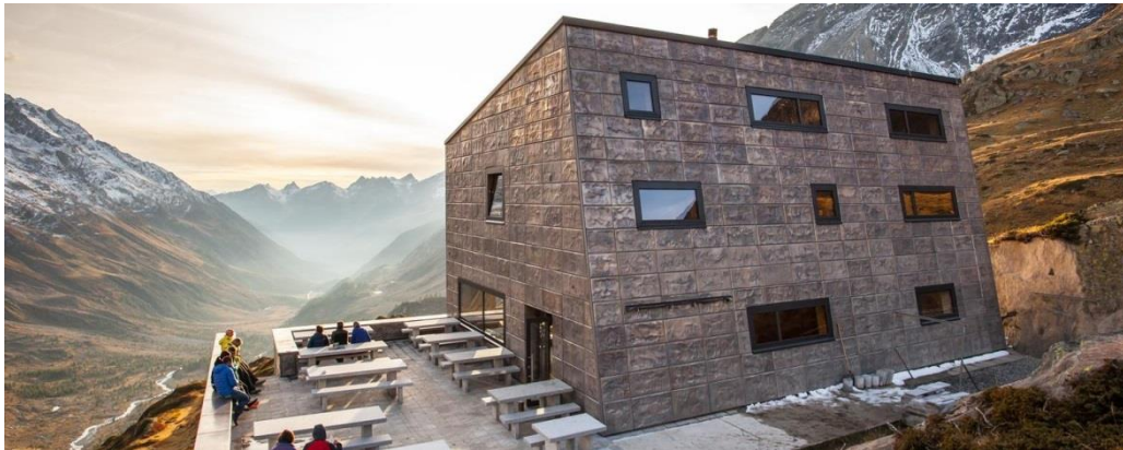
Figure 6. Lötschental, Switzerland, Cottage Anenhütte
