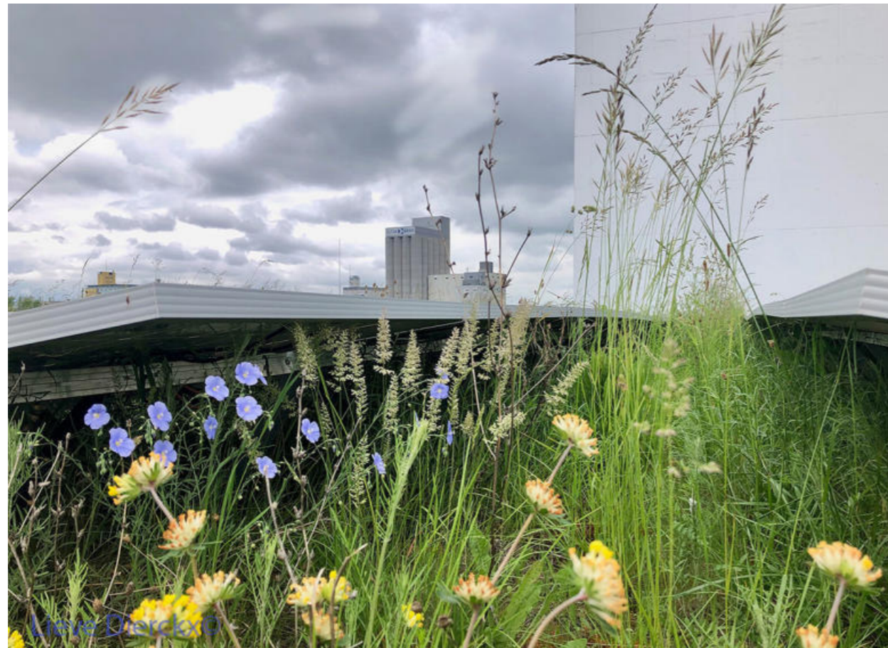
Figure 1: Roof of the shopping centre Stücki, Basel, Switzerland. Plant species rich extensive green roof with photovoltaic installation. Copyright: L. Dierckx
