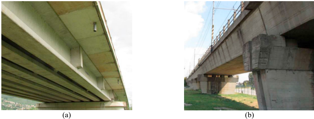
Figure 1: Typical spans for the two case studies: the railway viaduct with PRC girder beams deck, case study A (a) and the one with box girder PRC deck, case study B (b).
