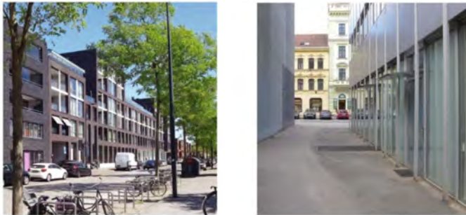
Fig. 2. Case 01: Ground floor visual permeability and the frequency of openings reinforce safety. Left: Amsterdam, 2018; right: Prague, 2020 (Photographs by Šárka Jahodová)
