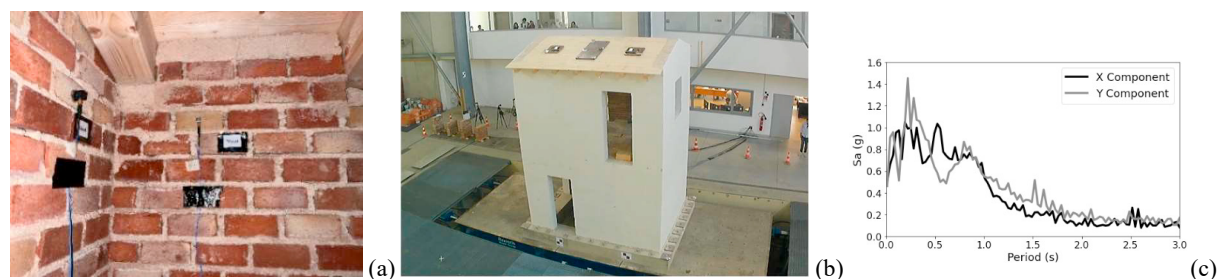
Fig. 5. (a) View of the sensors installed in the inner sides of the walls; (b) Overall view of the specimen in the shake table; (c) Response spectra of the reference input earthquakes.
