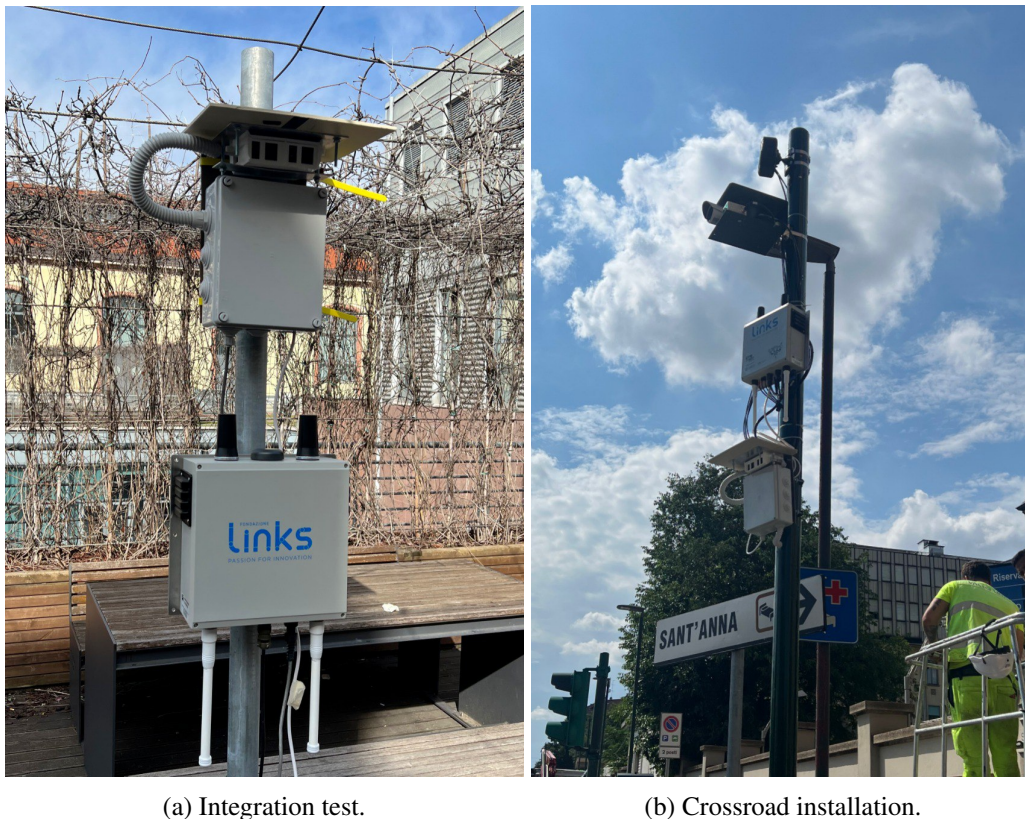
Fig. 2.7 Setup of crossroad experiment [5].
