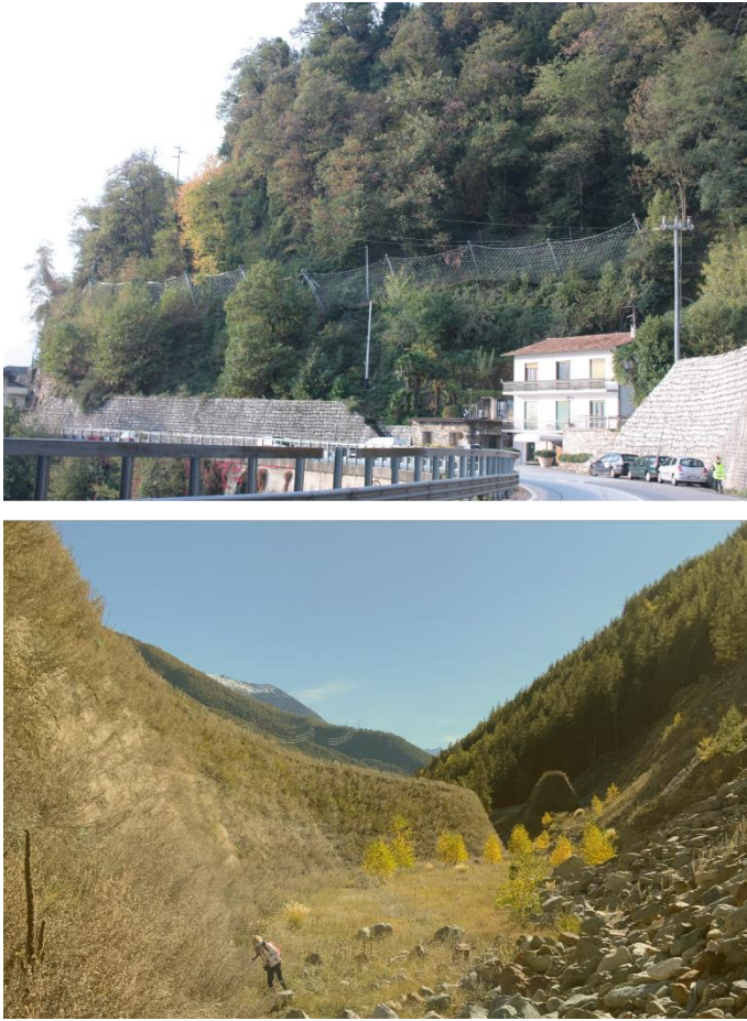
Figure 1. In the top, view of a rockfall net fence along a road. In the bottom, view of a rockfall earth embankment.
