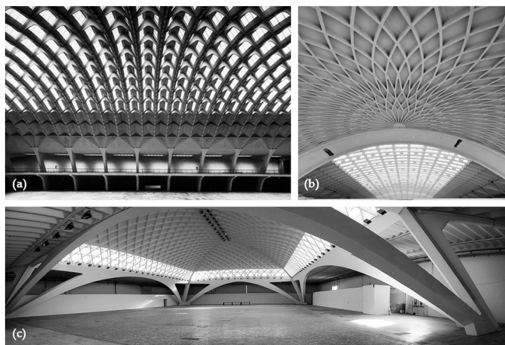
Figure 1. The wide and impressive reinforced concrete vaulted structures of the Nervi’s halls (photos from the archive of the conservation plan—Politecnico di Torino): (a) the wide undulated vault form pavillon B; (b) the semi-dome ribbed vault of the exedra, pavillon B; (c) the inclined arches from C pavillon.
