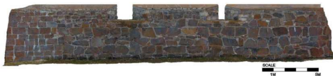
Figure 7. Orthophoto of Wall Section.
