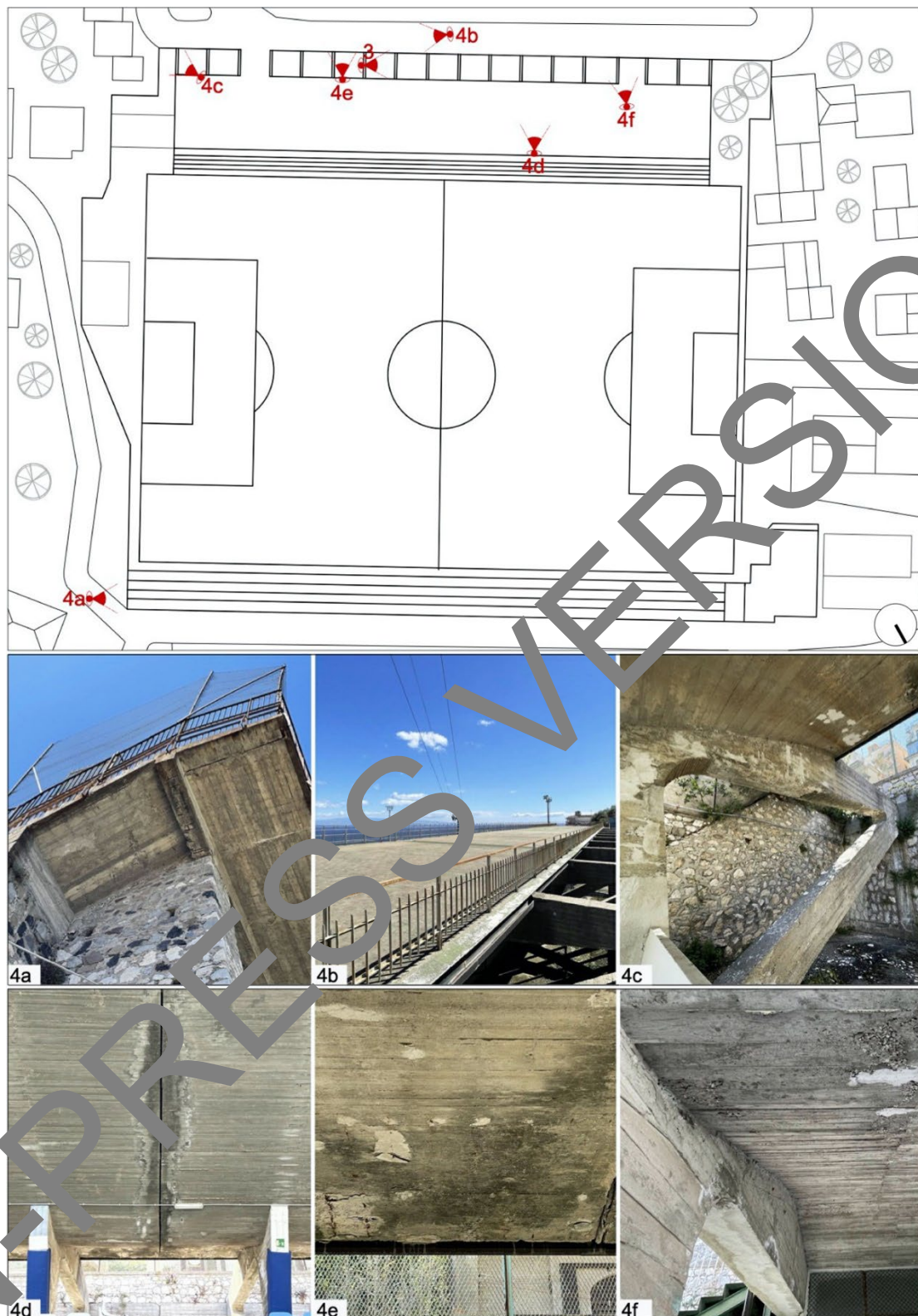
Figure 4 – Details of the degradation and location in the floor plan: (a) the north stand in structural decay, (b) the abandoned terrace, (c) aesthetic degradation from incorrect patching and vegetation, (d) degradation at the structural joint, (e) lack of concrete and spalling, (f) construction defects such as honeycombs - © 2021, Authors
