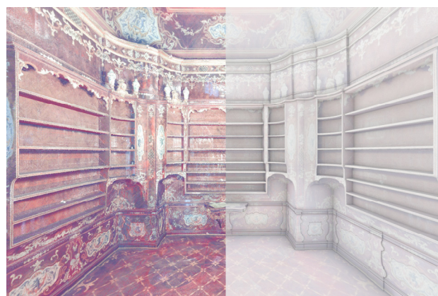
Figure 7. Comparison between photogrammetric survey and 3D model of Quirinale library (Modelling and editing: E. Pupi).
