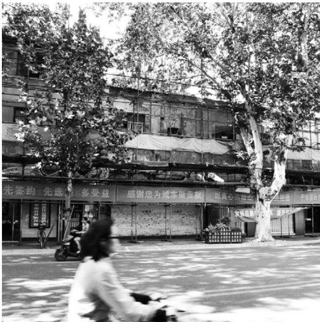
Fig. 04 - Red banners on building to be demolished in Taiping Nan Road
