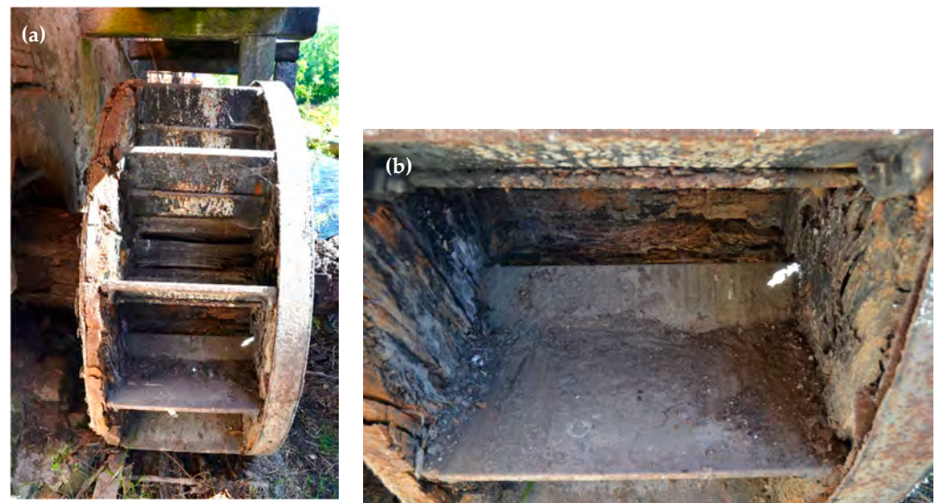
Figure 18. Details of water wheel #2: (a) front view; (b) shape of the blade.
