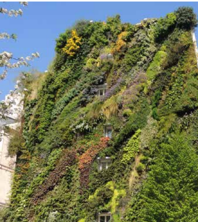
Figure 8. Continuous living walls system. Compact coverage of different plant species.
