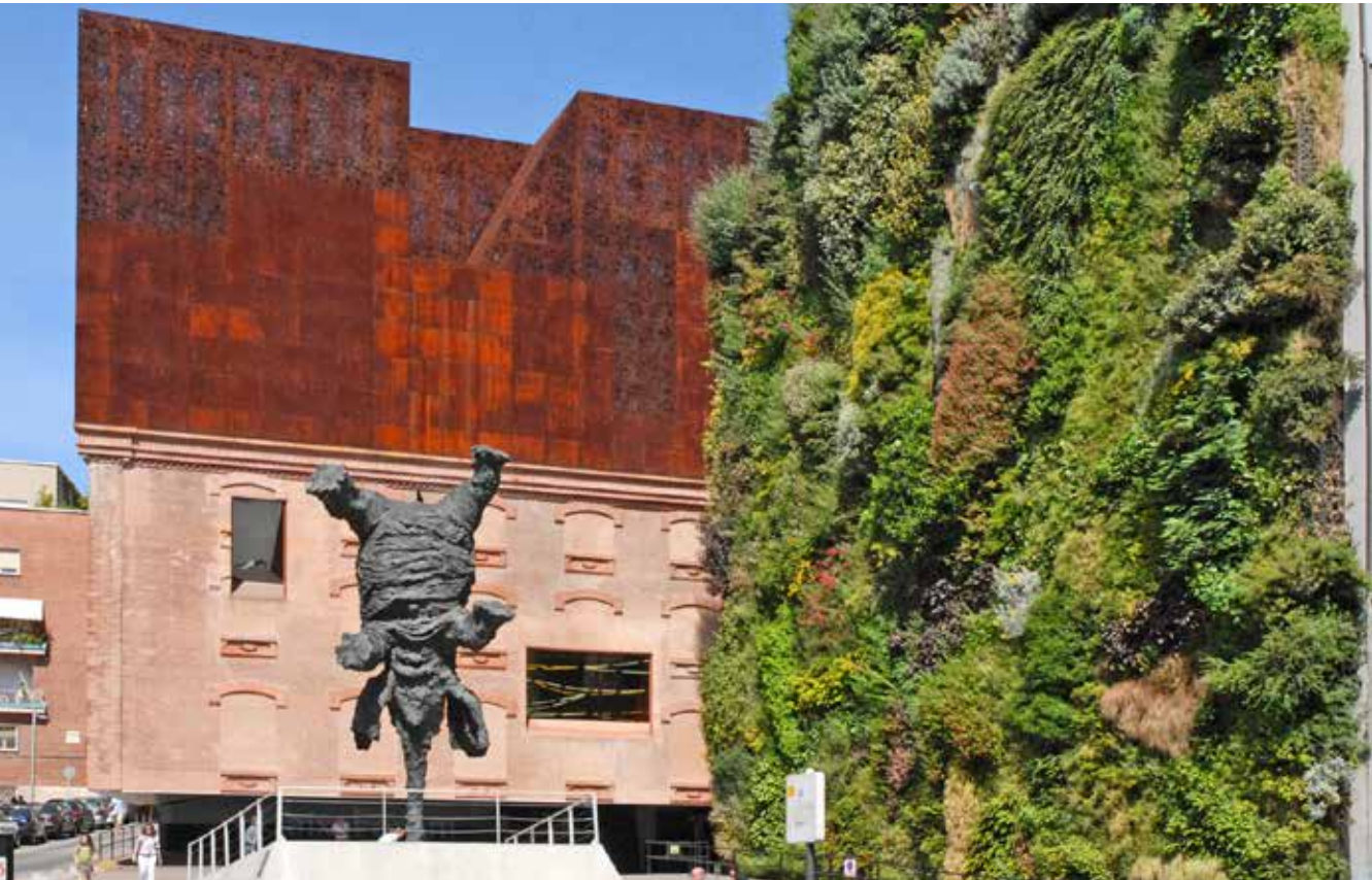
Figure 16. Caixa Forum, Madrid. Application of Le Mur Végétal system by Patric Blanc in 2001.
