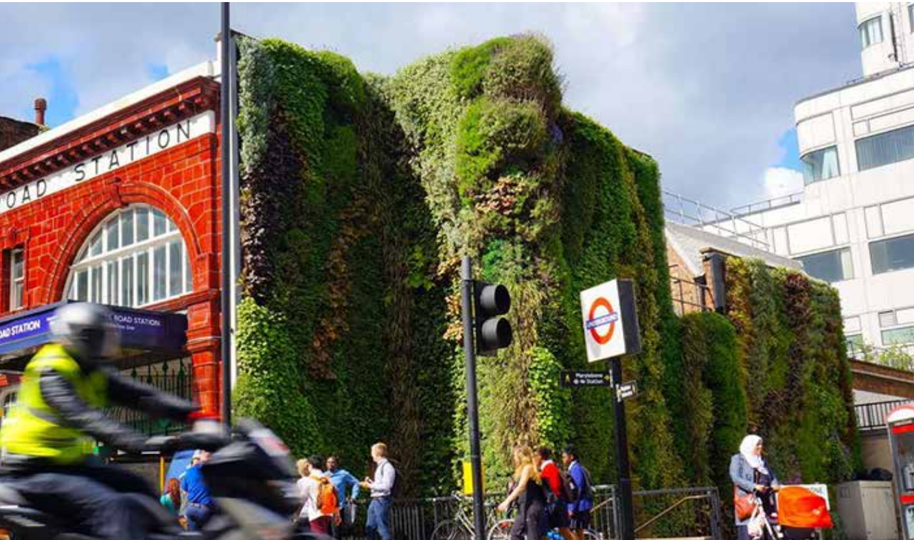
Figure 34. Biotope's green walls installation at the Bakerloo Line station in Edgware Road, London (UK).
