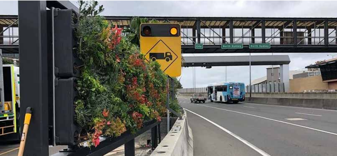
Figure 33. Junglefy’s green wall along a section of the Transurban Easter Distributor highway
