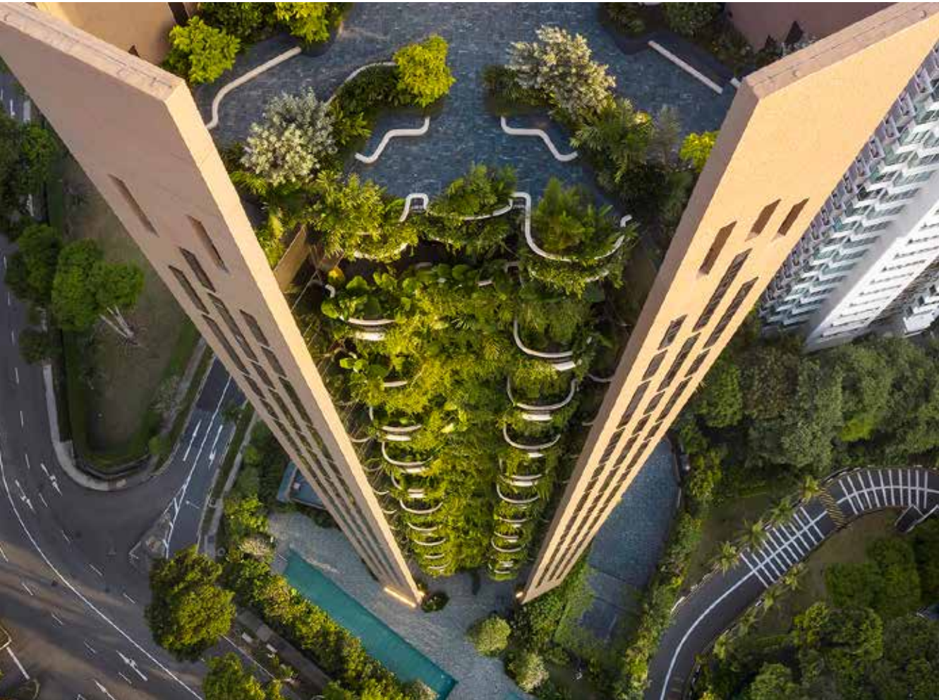
Figure 28. LUSH program. Systematic and highly technological integration of vegetation on the vertical development of the city of Singapore.
