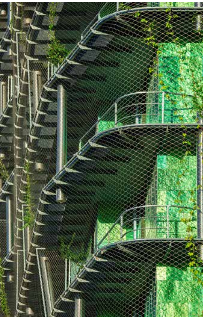
Figure 41. M6B2 steel cables structure.
