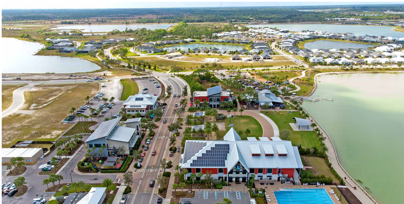
Fig. 3.37.1 Centro del Babcock ranch ©BabcockRanch
