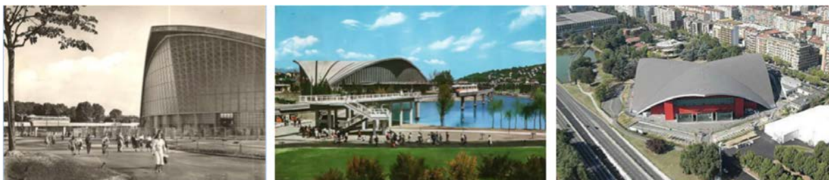
Fig. 5. Left and middle: "Palazzo a Vela" in its original version [13] and right its reuse by Gae Aulenti Architect (2003) [14].
