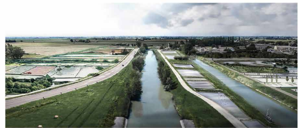
Fig. 9 - The Sant'Antonino case study. The water management systems are integrated in a park next to the Cona Hospital where wetlands and collective spaces hybridize with each other (elaboration by the Authors).
