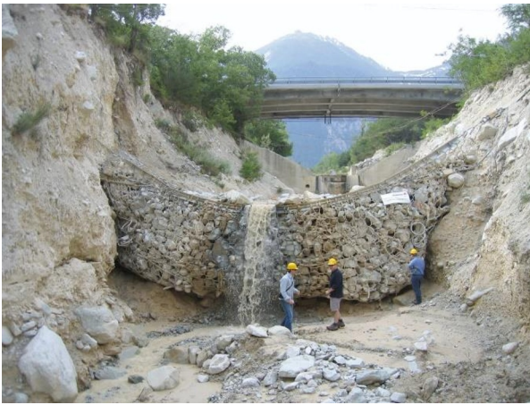
Fig. 1 Debris flow flexible barrier (Courtesy of Geobrug Italia)
