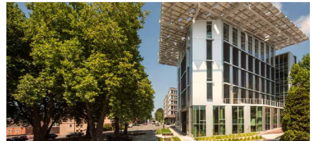
Bullitt Center, Seattle da: https://bullittcenter.org
