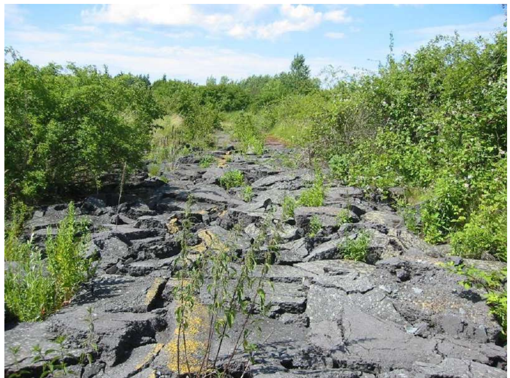
Figure 6. The airfield's impervious surfaces are broken up and gradually undergo spontaneous naturalization (credit: reproduced with permission from GTL Landschaftsarchitektur; photo: Werner Rose).
