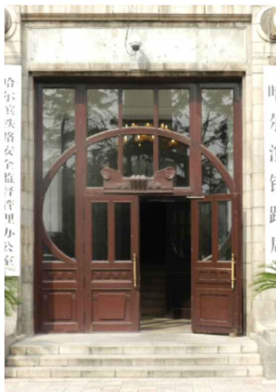
Fig. 1. Harbin (China). CER Management Bureau (1902), main entrance. Photo R. Tomborrino.
