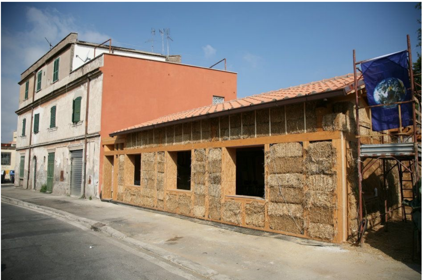
[SCh9] Figure 4: Straw bale house in Rome, Italy. Photo Credit: esbg2015 by Herbert Gruber
